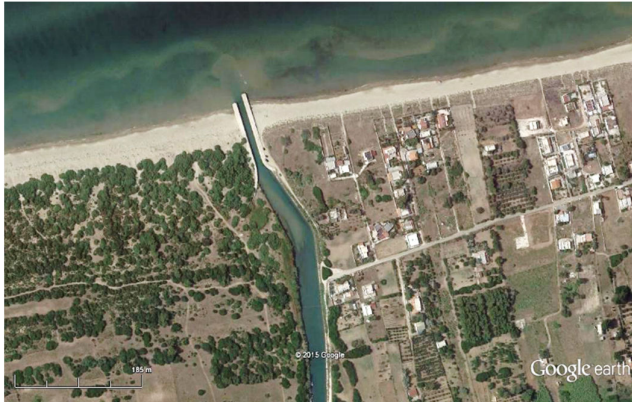
Constructed channel in Lesina, South Italy
